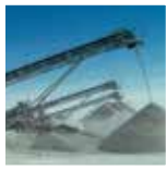
GRAVEL AND CONCRETE PLANTS
