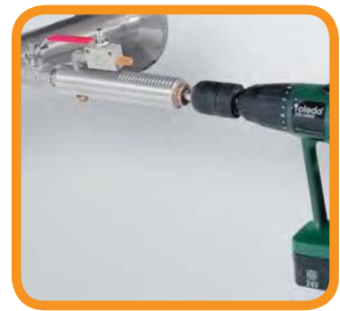
Drilling under pressure
